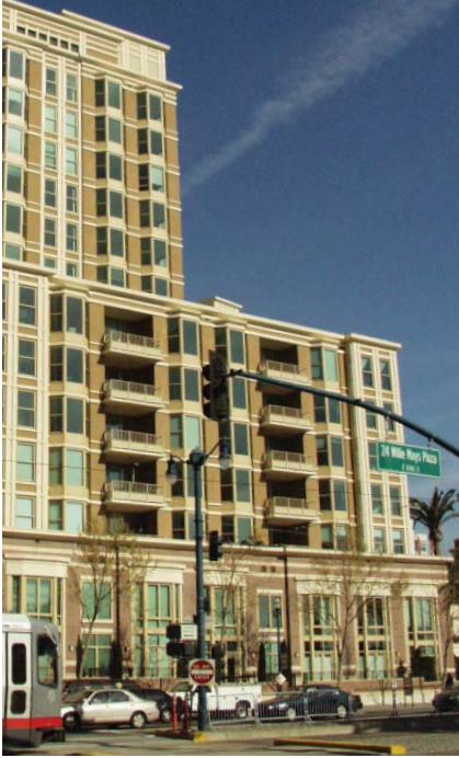
This building in San Francisco, CA gradually steps back from the street edge to ensure sunlight access to all units.
