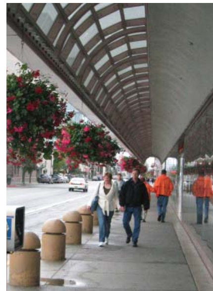
The canopy on the south-facing side of the Egan Center is an example of good northern climate design. Its transparency allows sunlight access, while sheltering pedestrians and preventing the build up of ice and snow.
