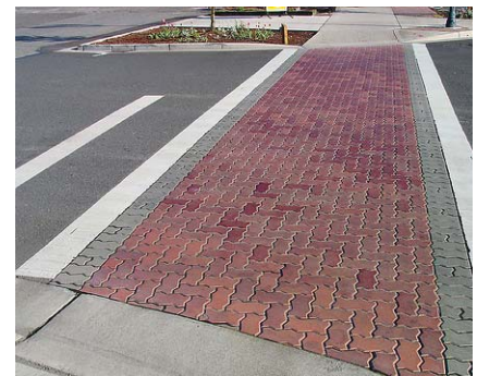
Raised intersections (middle left and right) or raised crosswalks (bottom left), or special material treatment (top and bottom right) at key pedestrian crossings will help distinguish the pedestrian zone, improve walking conditions and slow down through-traffic.
