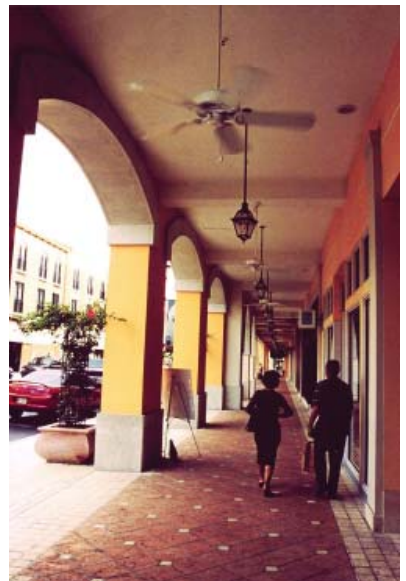
The arcades at right and above right feature high ceilings for openness, daylighting and ventilation. They are designed with aesthetically attractive colonnade forms and warm, light colors. Ceiling lighting and transparent storefronts provide evening illumination. Arcades can also include climate control features—such as fans in hot climates or heaters in northern climates.
