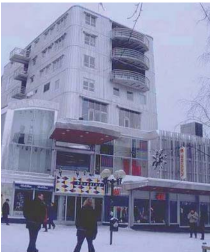
This building in Lulea, Sweden has a narrow east-west profile, a roof that slopes down toward the north, and a stepped façade that allows sunlight to reach neighbors for more of the year. Numerous facade elements break up the downward wind flow, lessening wind impacts at the street level.
