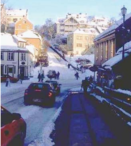
Heated sidewalks in Trondheim, Norway make pedestrian access safe and easy.
