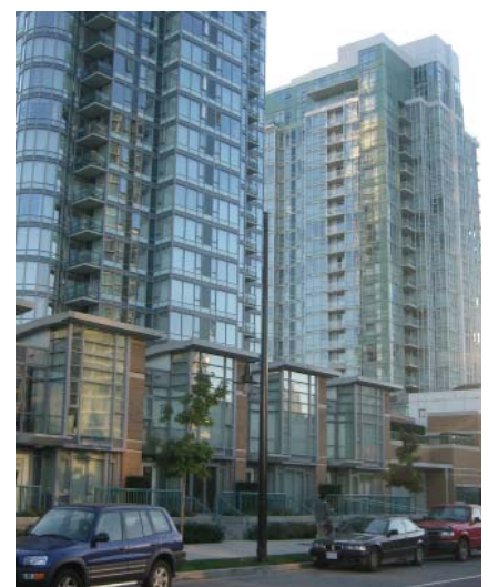
This high-rise construction in Vancouver, BC steps back from the street edge above the second floor.
