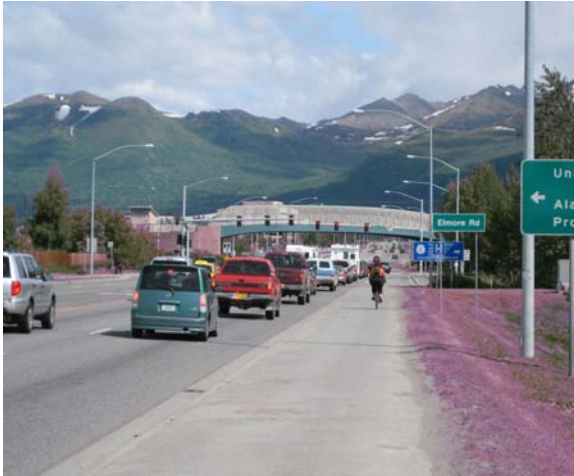
Back-of-curb pathway – Tudor Road
