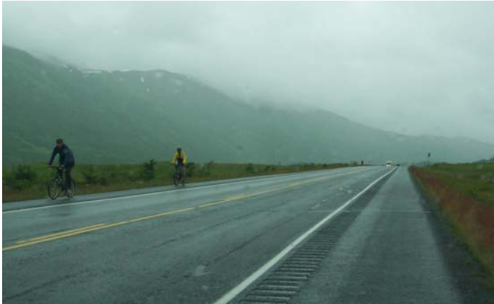
Rumble strips and bicyclists – Turnagain Pass
