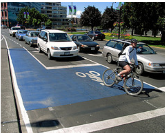
Bicycle box – for left-turning bicyclists
